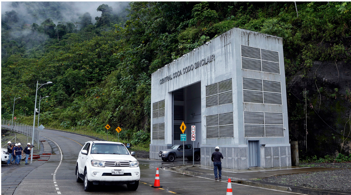
Outside view of the Coca Codo Sinclair hydroelectric power plant in Napo, Ecuador, on November 20, 2018.
